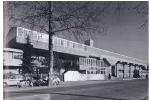
Figure Q15 Façade sud Image M.S.S.
