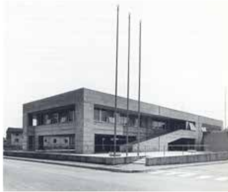
Figure P3 Façade principale Image P.E.A.
