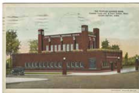
Figure S3 The People Savings Bank of Cedar Rapid, Iowa - L. H. Sullivan Image urbanremainschicago.com
