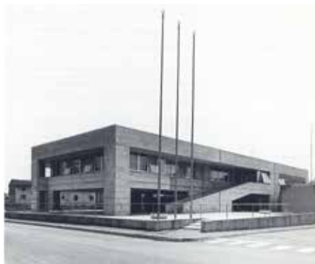
Figure P3 Façade principale Image P.E.A.
