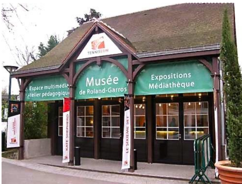
Figure 32 - Le Tennisium, 2015 - Source : Do Tours
