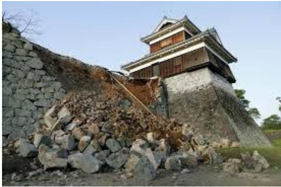
Photo 3: Kumamoto Castle damaged during the 2016 earthquake Source: Shinichi Saoshiro, 2016
