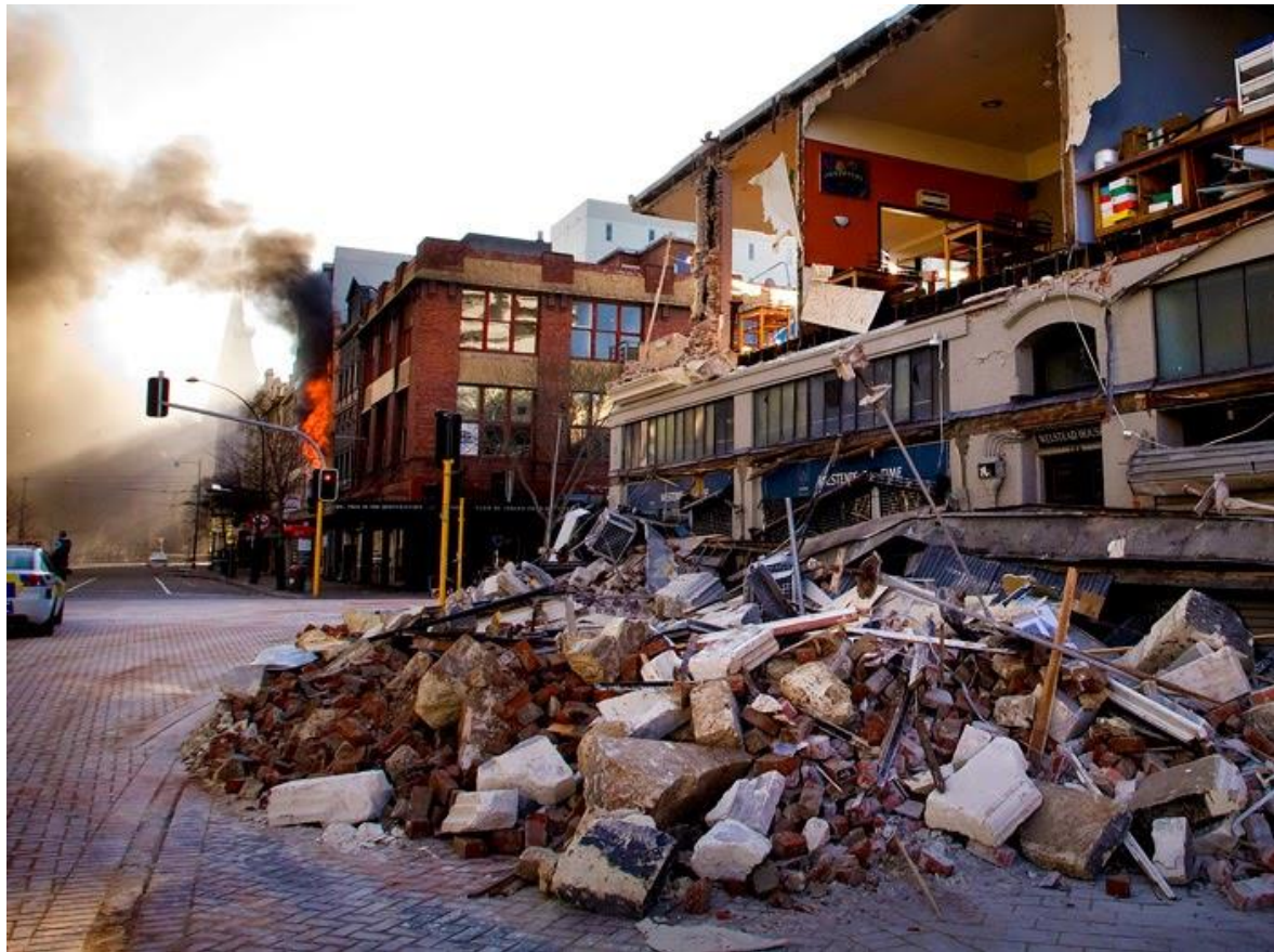
Photo 1: Christchurch earthquakes of 2010 Source : Blundell, S. 2018
