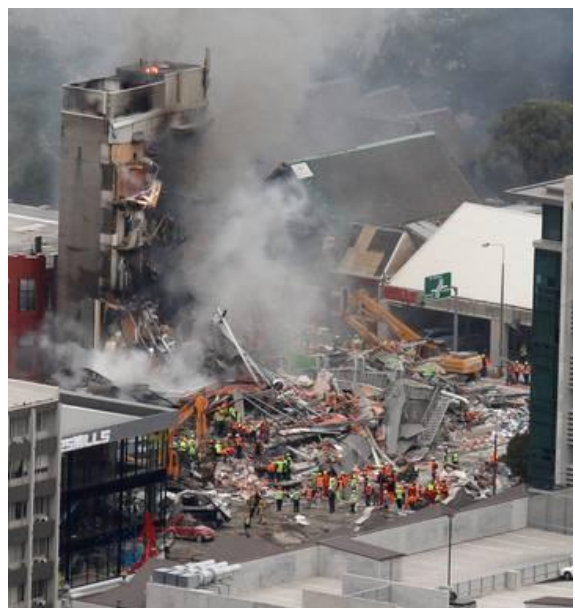
Photo 2: CTV building - Christchurch 2011 Source: Mark Mitchell
