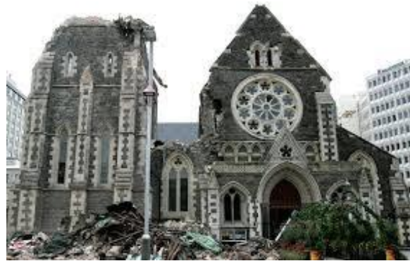
Photo 4: Christchurch Cathedral damaged during the 2010 and 2011 earthquake Source: Greater Christchurch, 2011
