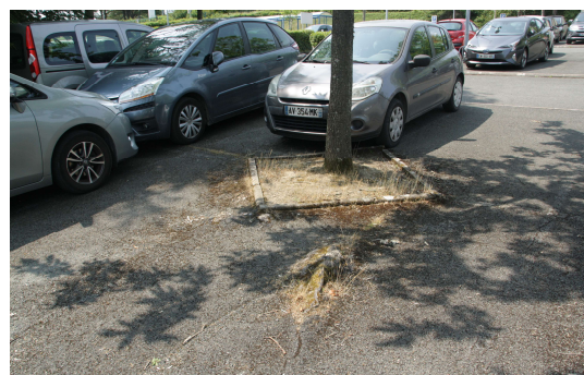
Figure 34 Des fosses de plantation insuffisantes, (Pethe, 2020)
