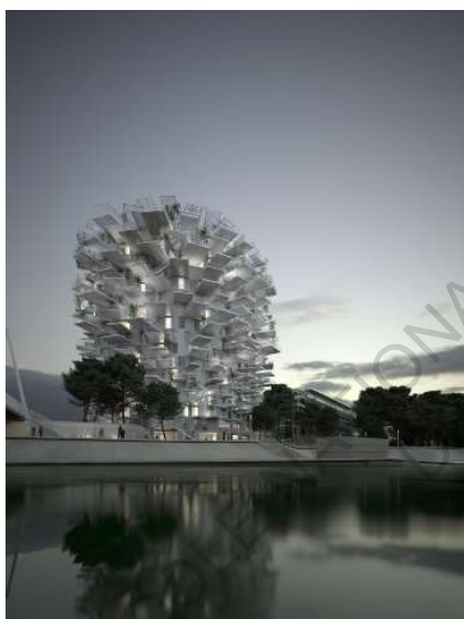
Fig. 108 Sou Fujimoto Architects + Oxo - Folie Richter, Montpellier - 2014
