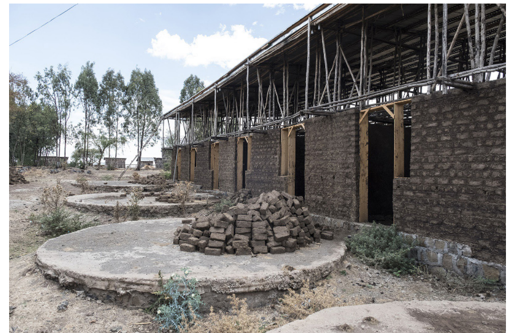
NESTown Project. Bura, Amhara. Chantier en cours de construction. Photo de NESTown.
