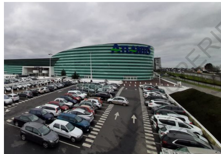
Centre-commercial Atlantis, St-Herblain, J.Sureau 2020
