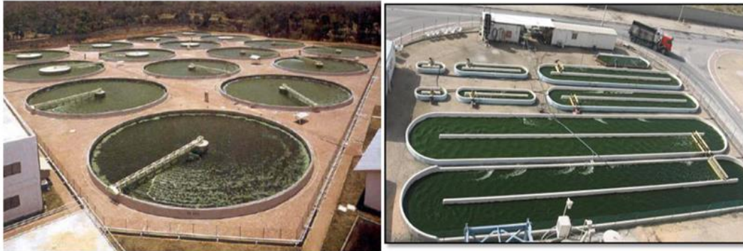
Figure 2 : Pictures of two types of algae tanks, circular tank on the left. raceway tanks on the right (Ben Amor, 2015).
