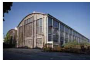
Grande halle SNCF
