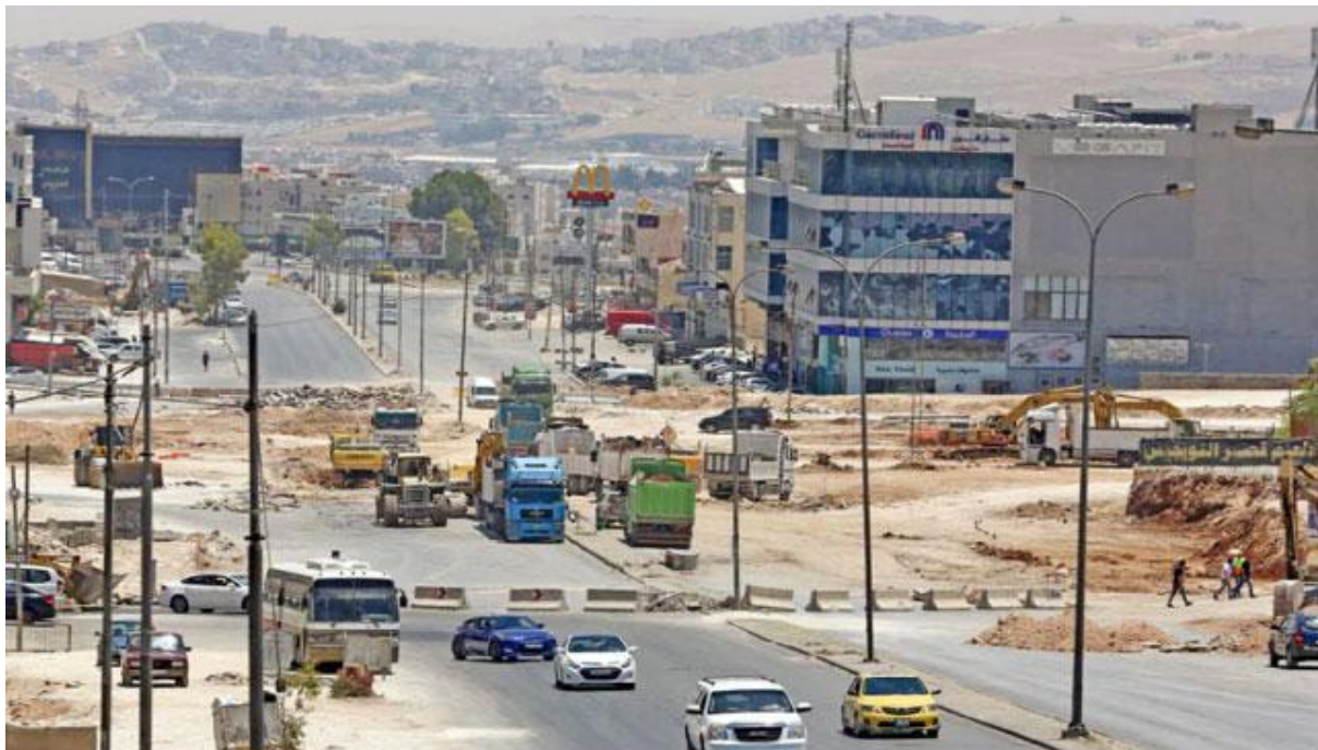
Figure 22: Constructions works on Tabrbour intersection, Source: Jordan Times, 2019
