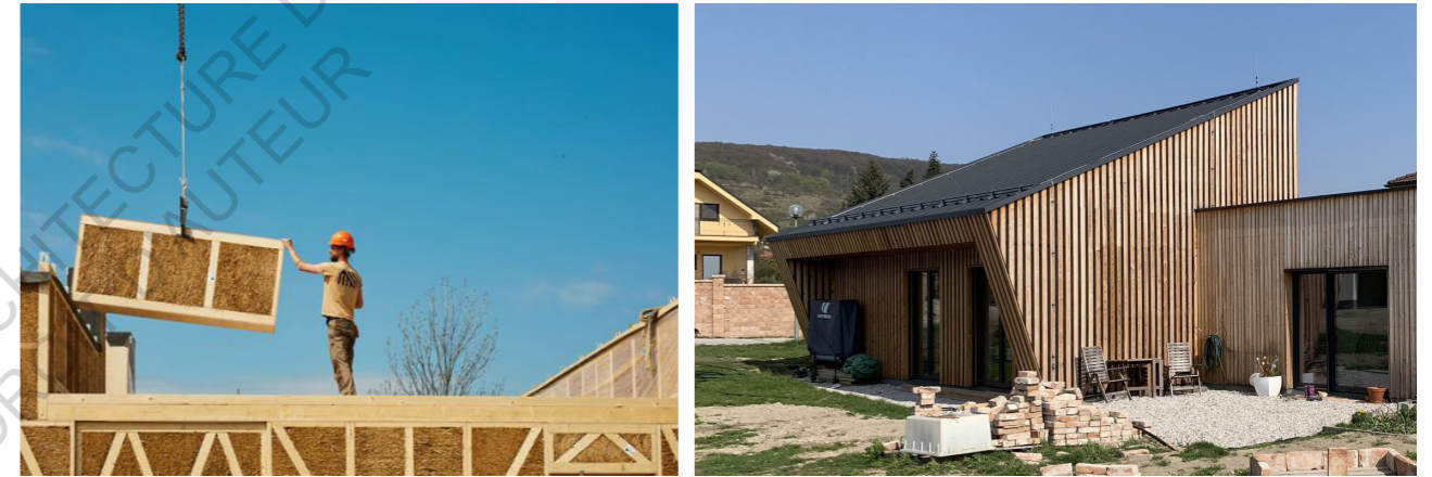
EcoCocon panel being assembled and a completed project, the Solar Kit House.
