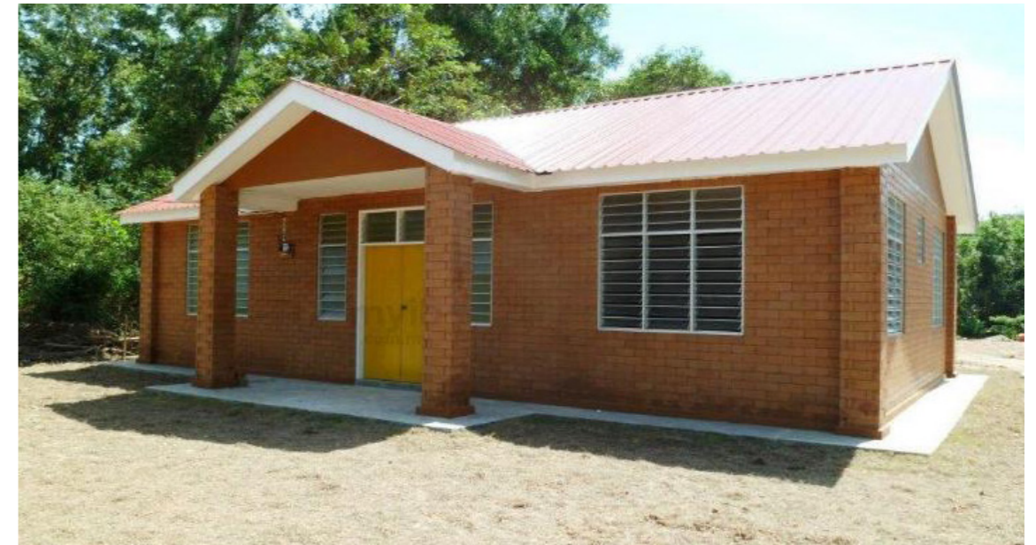
A Malaysian Interlocking Bricks column being reinforcement by steel bars and a completed public housing.
