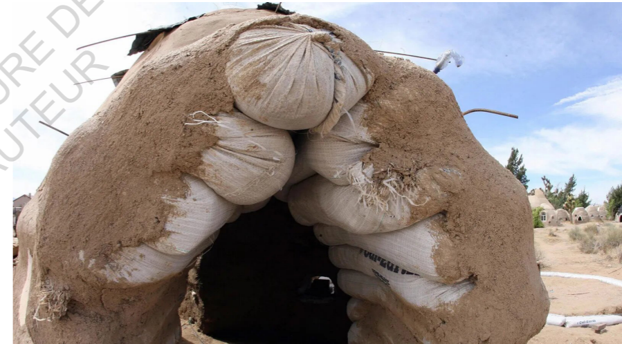
Superadobe-filled bags being covered with another earth mixture, next to finished superadobe houses at the Cal-Earth Institute
