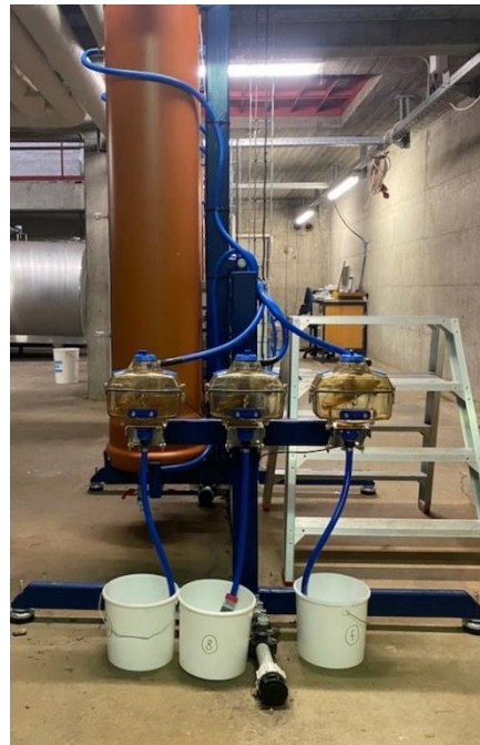
Figure 17: Tipping bucket flowmeter and water sampling of reactor (picture from Lars Elsgaard)
