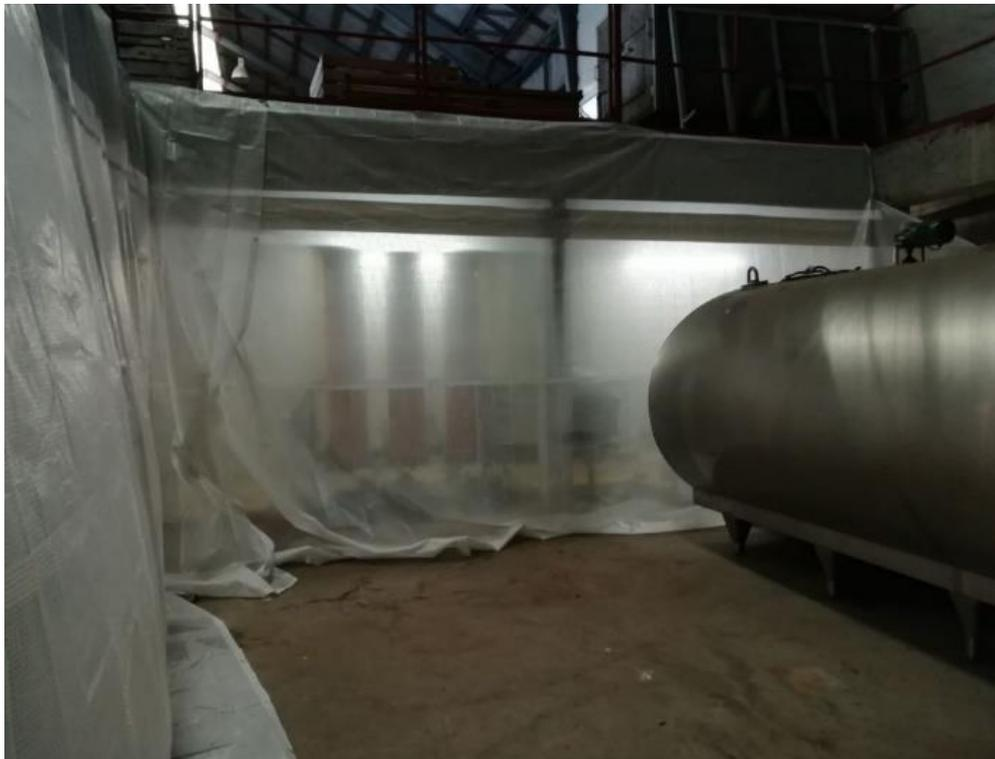
*Figure 22: Thermal isolation system*
