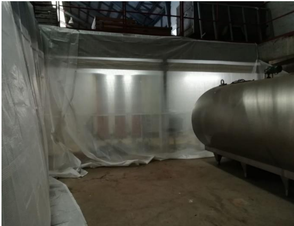
Figure 22: Thermal isolation system
