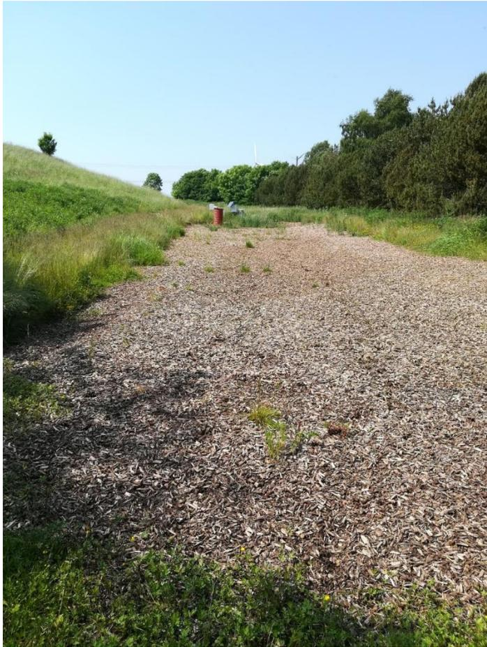
Pilot scale woodchip bioreactor or sub-surface constructed wetland
