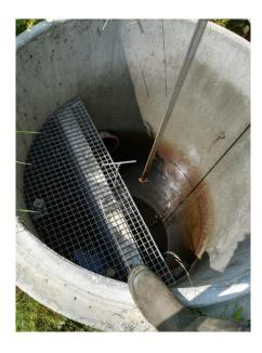
Subsurface draining system leading to the woodchip bioreactor
