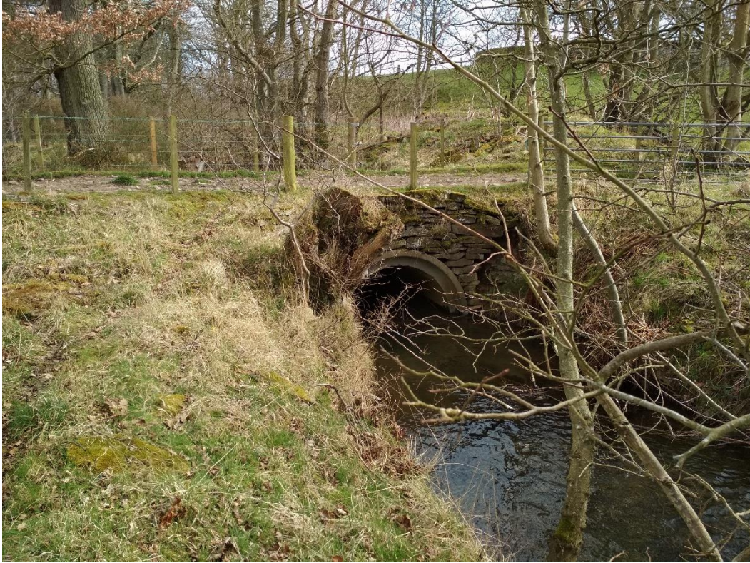
Figure 42 : south bridge from upstream, taken on the 1st april 2019
