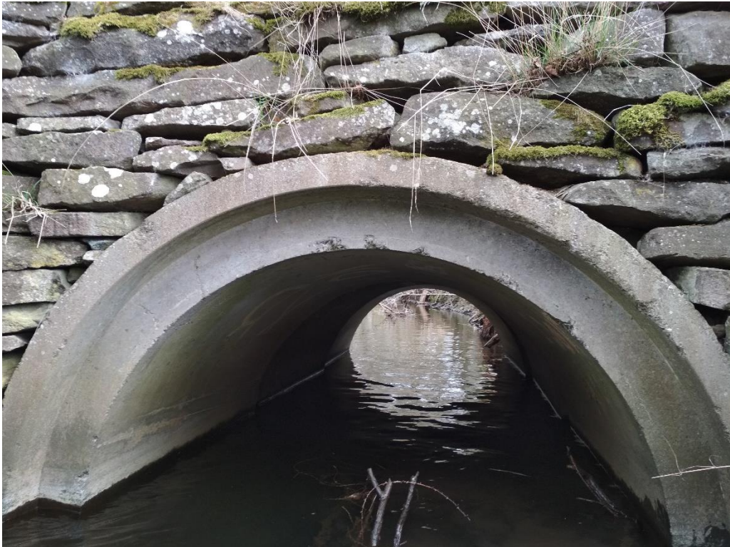
Figure 2 : south bridge from upstream, taken on the 1st april 2019
