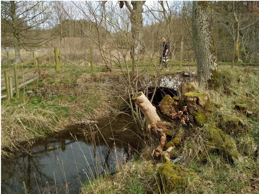
Figure 43 : north bridge from upstream, taken on the 1st april 2019
