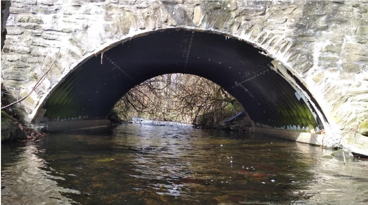
Figure 1 :view from downstream, taken on the 1st april 2019
