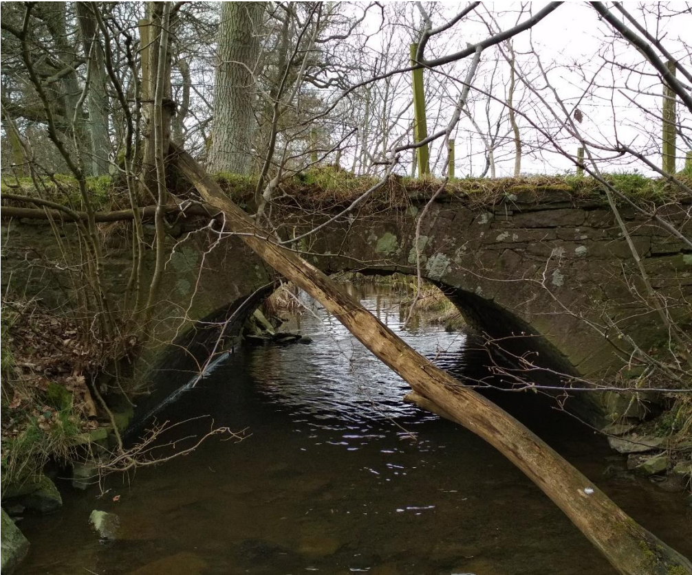
Figure 1 : north bridge from downstream, taken on the 1st april 2019
