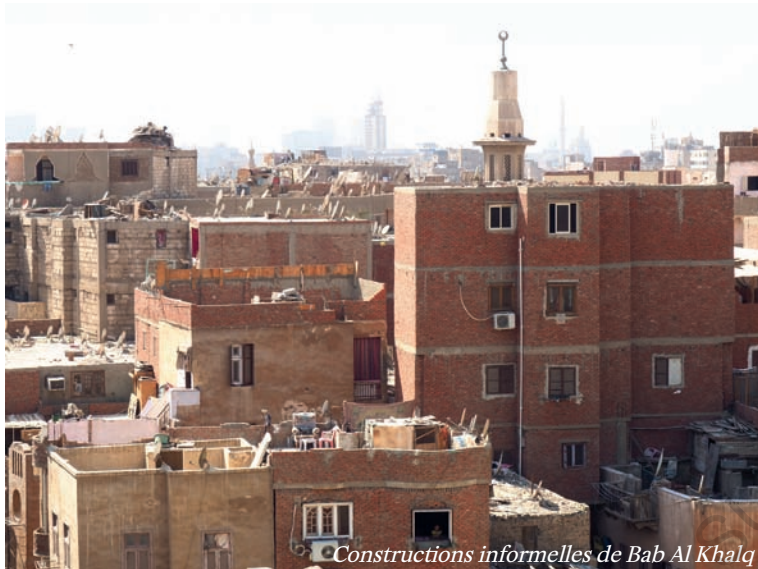
Constructions informelles de Bab Al Khalq
