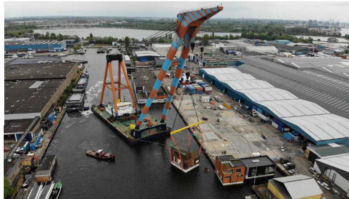
Fig 60 : Assembly of the modular homes.
