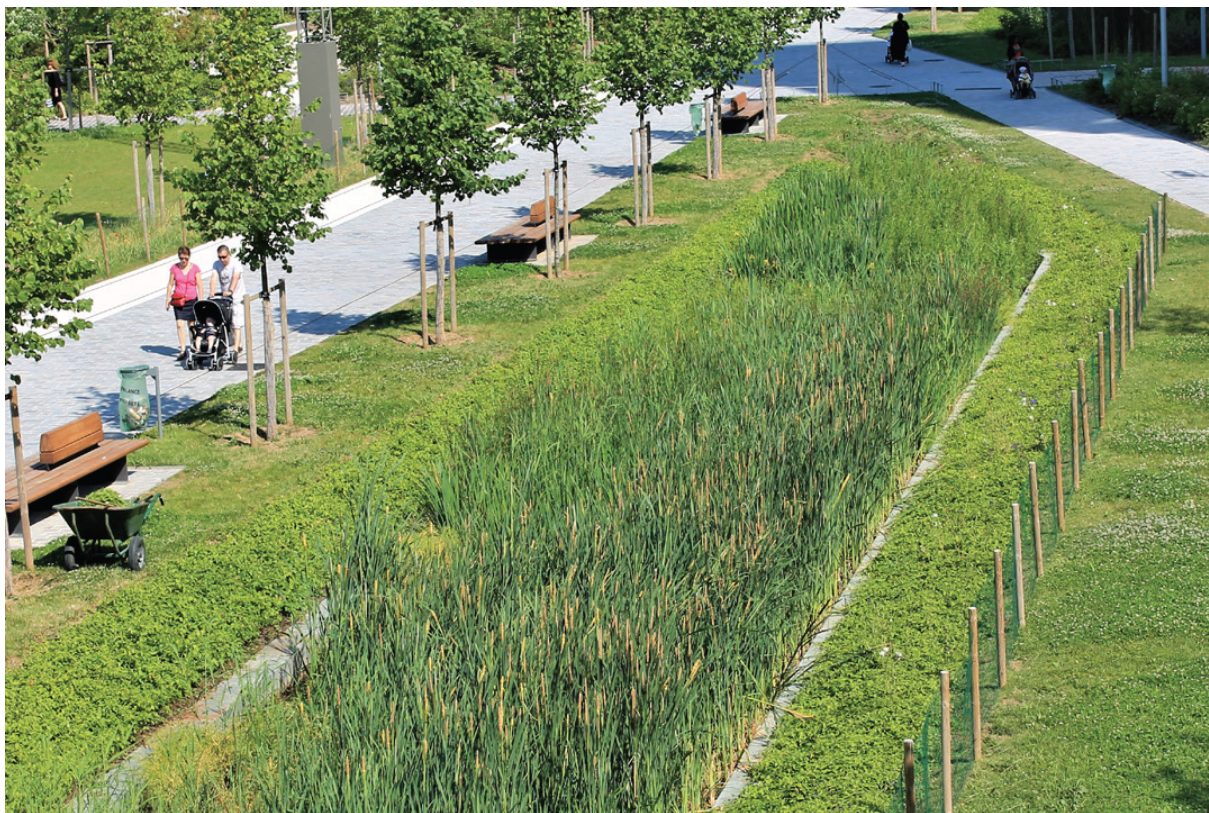
Reference image - Green collection and storage ditch - Martin Luther King Parc, Clichy Batignolles (ATM, 2021)
