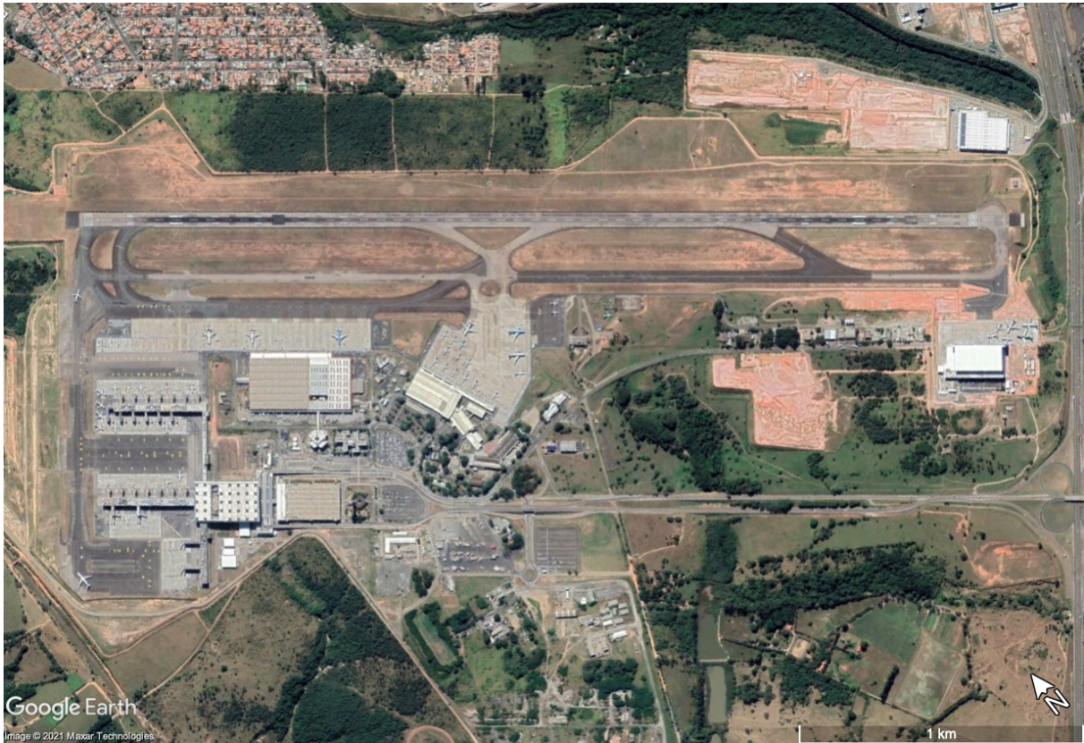
Figure 2 VCP airport site from the top Source: Google Earth
