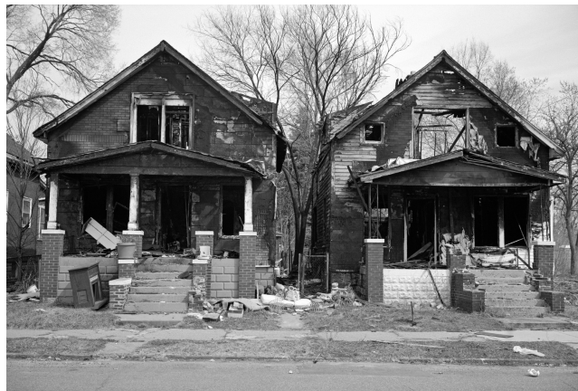
Illustration 1. Foreclosed homes in Detroit, Michigan. Photo from Bruce Gilden's Foreclosures (2013).
