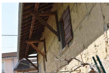
Consoles bois Phot. Magali Delavenne IVR84_20220100216NUCA
