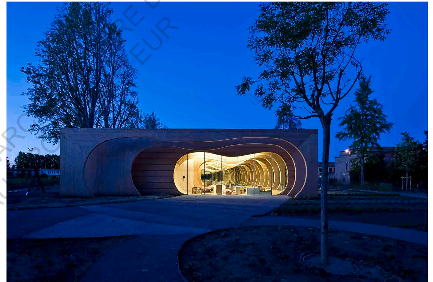
fig. 38 : crèche de Guastalla / Mario Cucinella Architects. Image © Moreno Maggi
