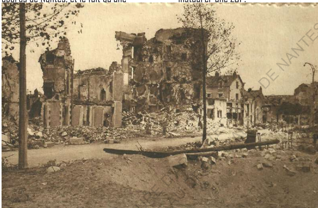
Destruction du quai Malakoff - Geneanet.org
