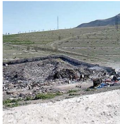
FIGURE 41: DECHARGE A CIEL OUVERT (81)
