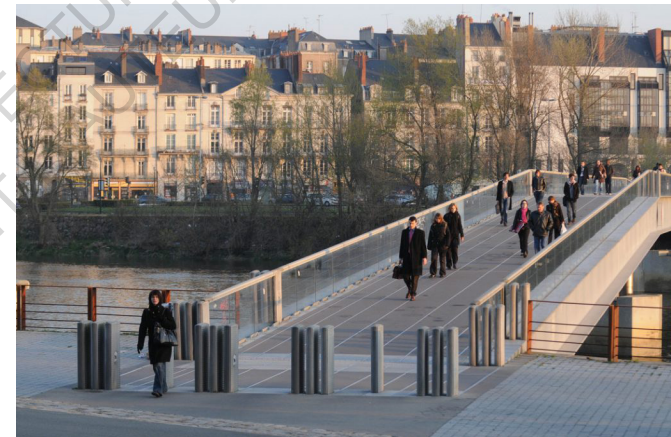
Figure 25. Passerelle Victor Schoelcher, Nantes, 2001 © Samoa
