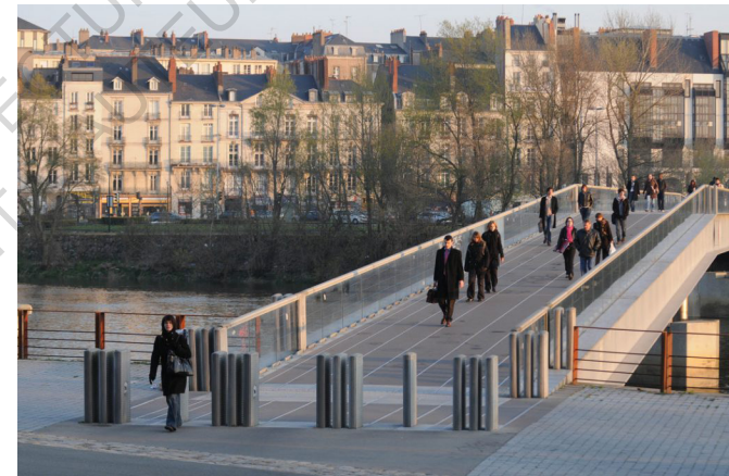
Figure 25. Passerelle Victor Schoelcher, Nantes, 2001 © Samoa
