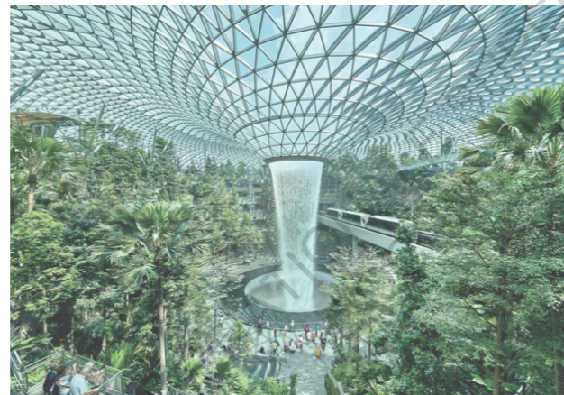
Jewel Changi Airport, Safdie Architects, Singapour
