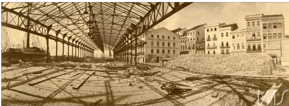
Figure 17 - 1910 picture by Francisco du Bocage showing warehouses being built in the neighbourhood of Recife.
