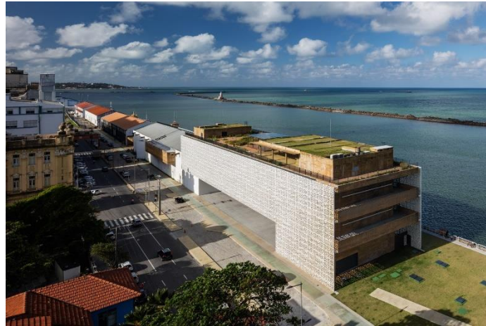
Figure 46 - Cais do Sertão Museum seen from above.
