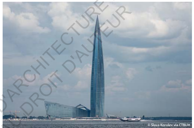
Lakhta Center - St Petersburg - 2020 - RMJM - 462m
