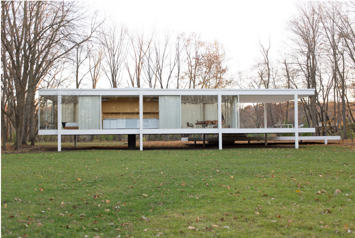
Figure 14, Farnsworth House (Illinois) 134
