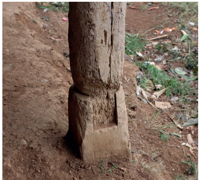
↑ Intelligence constructive locale
