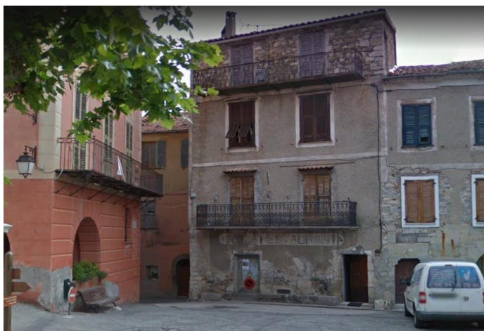
Figure 45 : Logement vacant, Utelle- Source : Streetview
