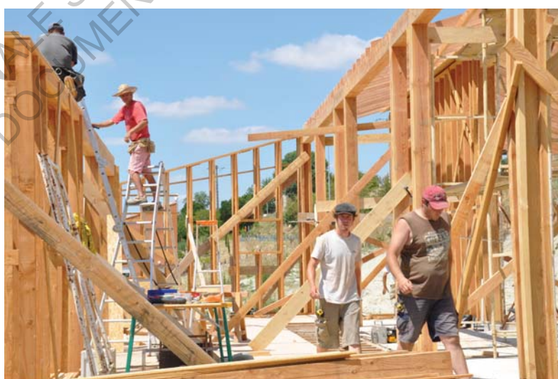
Figure 20: Pose l'ossature
