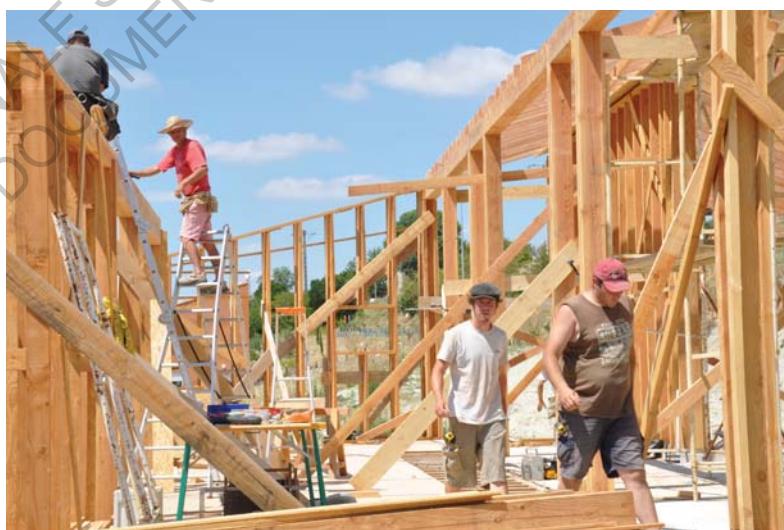
Figure 20: Pose l'ossature
