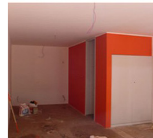
Fig.57: transformations de conteneurs.
