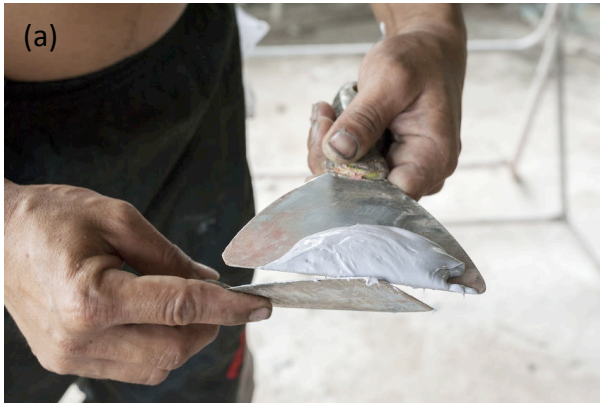
Figure 2 : (a) Mélange du mastic. (b) Application du mastic.
